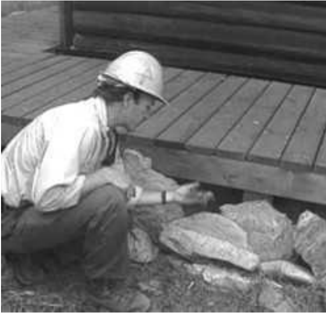
△ FIGURE A.17.1.8.3(a) Leaf Litter and Needles Collect in Small Spaces. (Courtesy of Firewise Communities Program. Photo by G. Johnston.) [1140:Figure A.24.3.4.3(a)]
